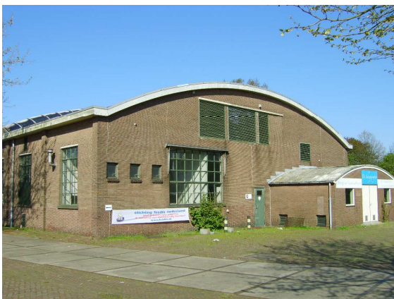
Fig.1: Barrel vault, workshop former Military complex, Woerden, The Netherlands.
