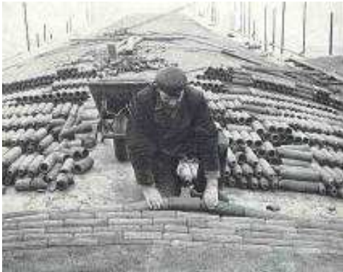
Fig. 6: Construction of a barrel vault [6].
